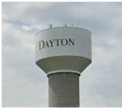
Figure 1. Name sign on existing 500,000-gallon composite tank
